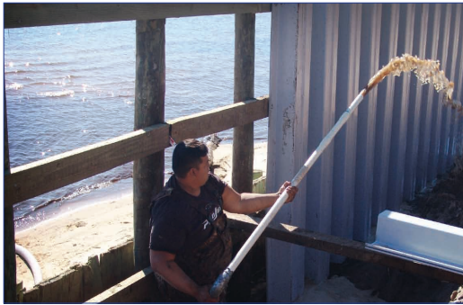
A water jet is often used to drive the vinyl piling into granular soil. In the above photo, you see a drive guide is used which provides a firm surface to drive the sheets plumb and straight.
