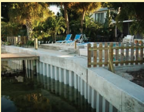
(Left) This canal front Florida homeowner selected the EverLast Vinyl 4.1 Series with a concrete cap.
